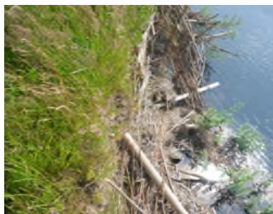
Pictures above showing steep bank with little or no re-profiling, narrow terraces, vertical posts too short and few live stakes all contributing to partial failure.
