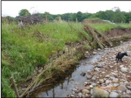
Figure 7: Details of willow stakes and rods installation
