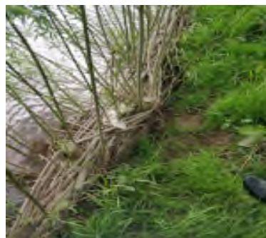
Pictures above showing willow spiling with very strong growth after 8 months (left). Live white willow vertical posts and low gradient bank (right).
