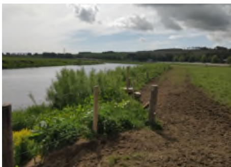
Pictures above showing willow spiling with very strong growth after 8 months (left). Live white willow vertical posts and low gradient bank (right).
