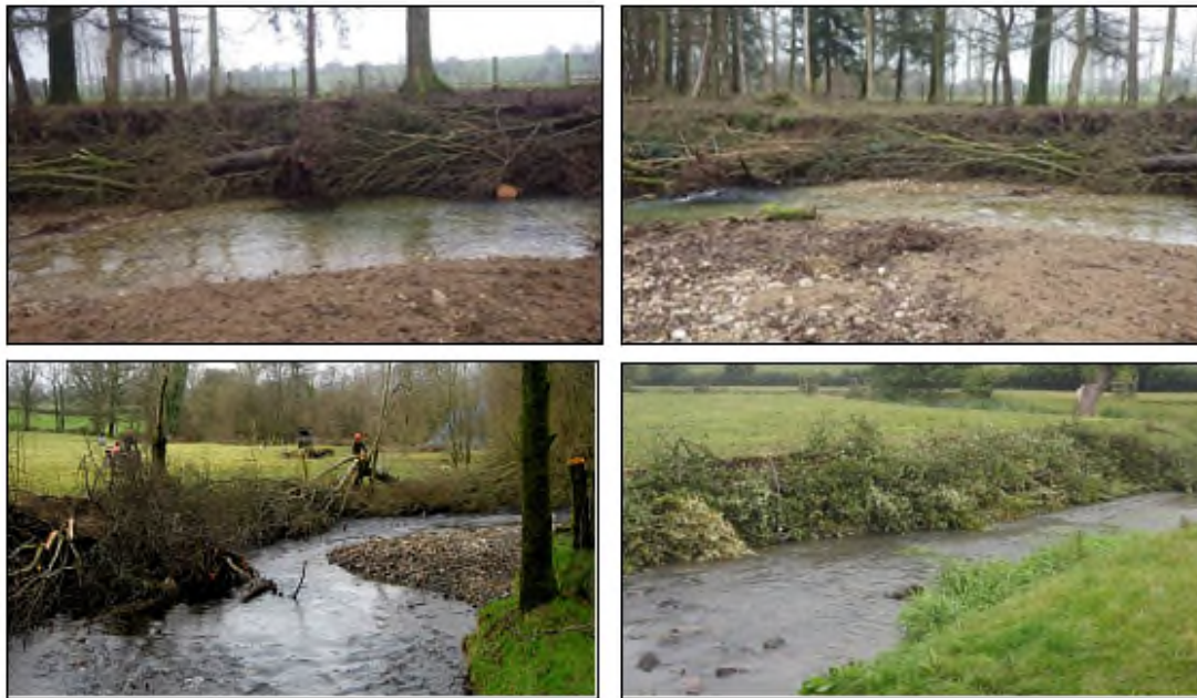
Figure 11: Examples of large wood used for river bank protection
