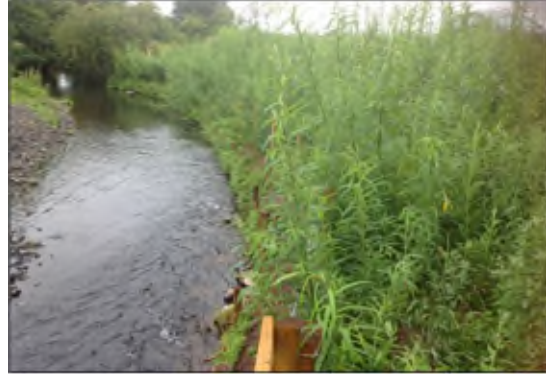
Figure 5b: Terraced willow spiling one year later, viewed from the opposite direction to Figure 5a. Note the complexity and roughness of the bank compared to that in Figure 5a
